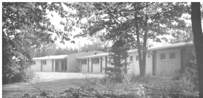
Motel built at the entrance of Carousel Mountain, ca. 1964
