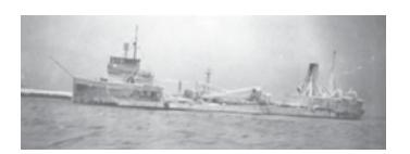
The *Burlington* was built in Chicago by the Chicago Ship Building Company in 1897. Her original name was the *Minneapolis*. She had a length of 238 feet, with a beam of 42 feet, a gross tonnage of 2,029, and net tonnage of 1,222. She was steel-hulled and laid out in the traditional bulk freighter style. In 1915, the vessel was sold to Shawmut Steamship Company in Boston, Massachusetts.
